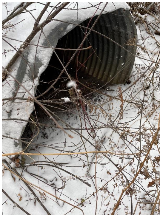
Photograph of SW-23 taken in December 2022
